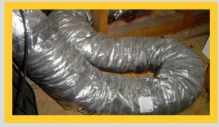
These large-diameter, wire-reinforced ducts can be used in long lengths, and have enough flexibility to snake around obstacles. Flex ducts are popular in attics and in any cramped space.
