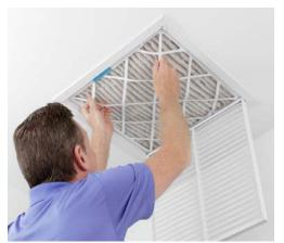
3. Identify the air conditioner filter size: A number or size should be printed on the edge of the existing filter. The replacement filter needs to be an exact match in order to fit correctly.
