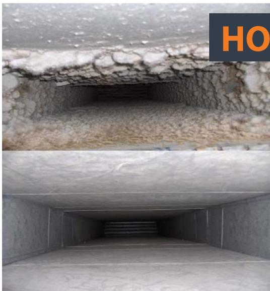
The most effective method of cleaning of air ducts is through "Source Removal." This requires a contractor to place the system under negative pressure through the use of a specialized, powerful vacuum. While the vacuum draws air through the system, devices are inserted into the ducts to dislodge any debris that might be stuck to interior surfaces. The debris are pulled into the vacuum and removed from the system and the home.
