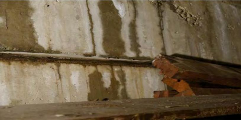
If there is puddling or flooding in your crawl space, then water is probably getting in through a crack, faulty window well or leaking from a pipe. Tracing the source of the water should be easy because it often leaves staining where it has run down a wall or out of a crack.
