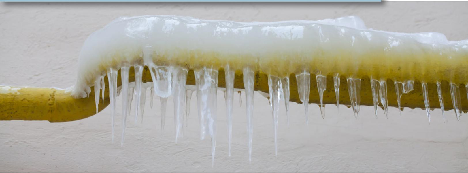
Homes in northern climates are built with their water pipes located on the interior of the building, which protects the pipes from freezing and subfreezing weather. Extreme cold weather and holes that allow cold air to come into contact with pipes can lead to freezing which can lead to bursting.
