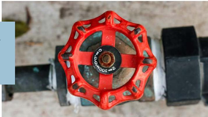
Above is an example of a water shut off valve, typically found in warmer climates. This valve will turn off the water to the entire home or building.
